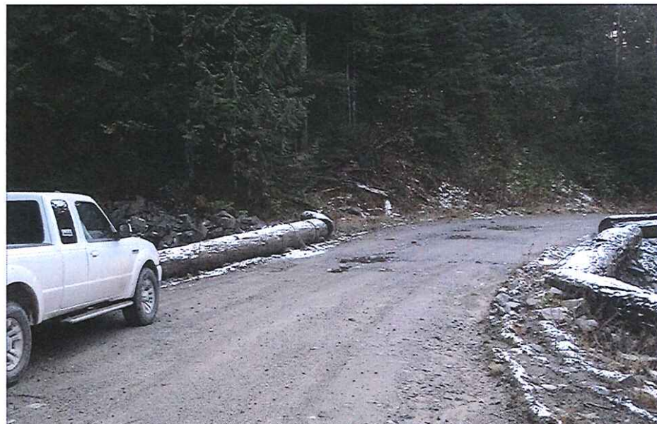
CK2455 Approach Left Bank
