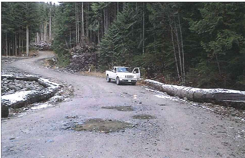
CK2455 Approach Right Bank
